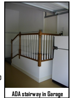
ADA stairway in Garage
