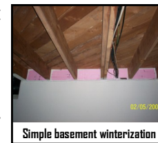
Simple basement winterization
